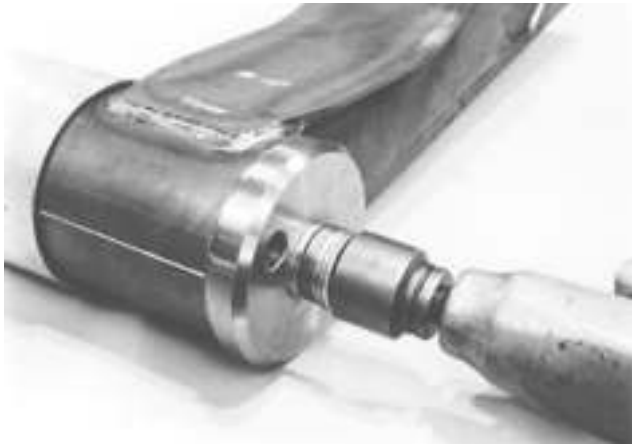
Figure 40: Installing bushing with impact wrench
